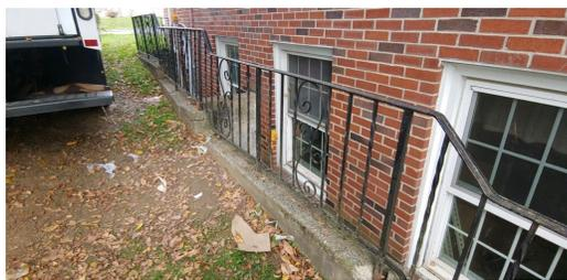
includes removal of the iron railing and the damaged portions of the wall, adding pipes for drainage, rebuilding the block wall, excavation for the new driveway, and paving. The approximate cost is \$23,650.
